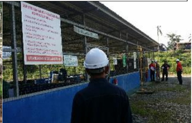
Scheduled Waste store and shower/eye wash facility in Mayvin Palm Oil Mill.
